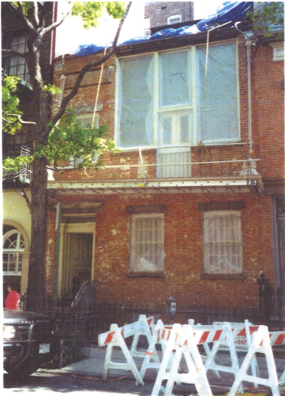
Façade during Adami restoration showing brick after cleaning and before repointing. Windows not yet replaced in this picture. Taken in 1997.
