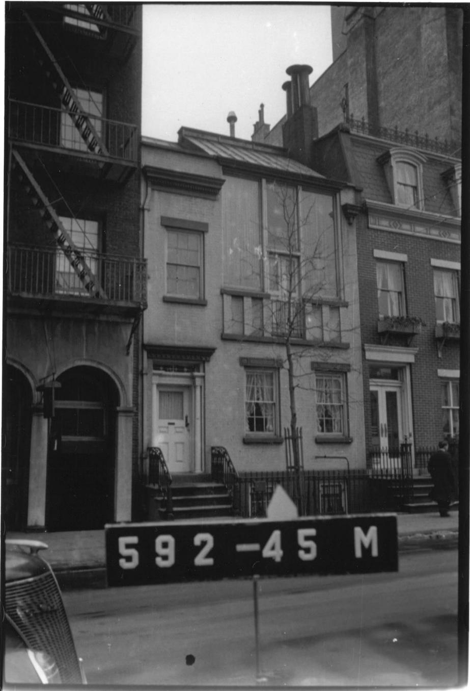
Tax photo circa 1940 showing roof leaders attached to cornice molding. Note extension of façade wall to form parapet on either side of the studio windows.
